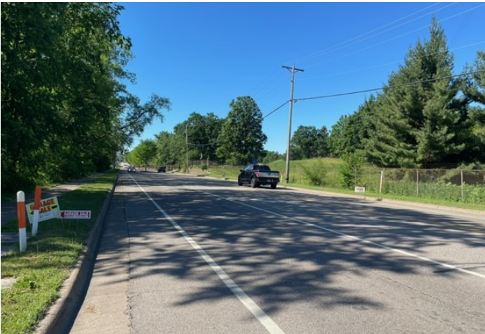
South view of Cleveland Avenue North.
